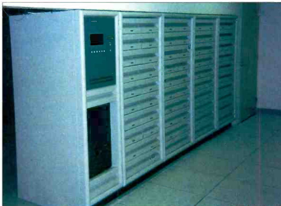
The Harris PT40CD DTV transmitter at WPLG-TV, Miami, gives 40kW peak and 10kW average power.
