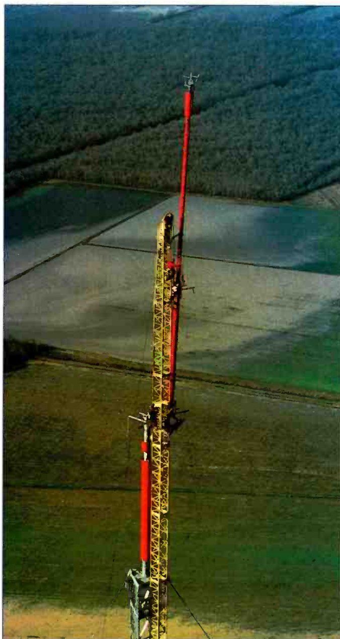
Photo of the installation of a 17-ton Dielectric traveling wave antenna on the nearly 2000-foot KNOE-TV tower near Monroe, LA. Photo courtesy LeBlanc Broadcast.
